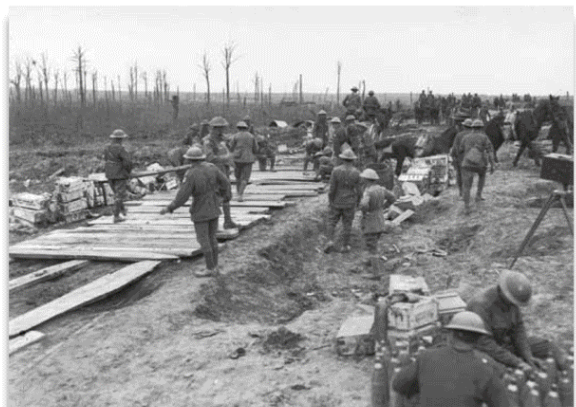
A Pioneer Battalion building a wagon track from planks of wood (note the desolate countryside).
